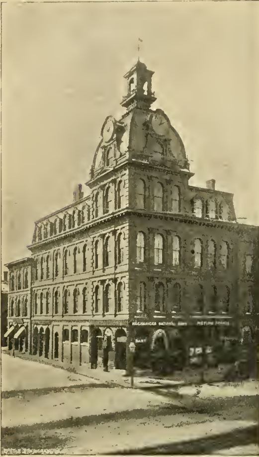
BOARD OF TRADE BUILDING, NORTH MAIN STREET.
